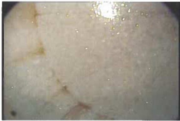
0:58 Typical view of roof plates
