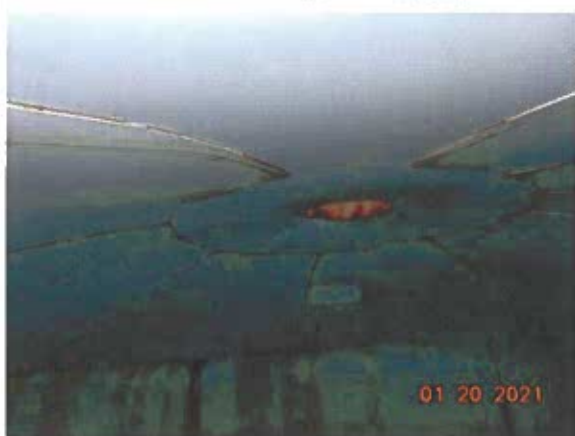
#21 Interior view of roof
