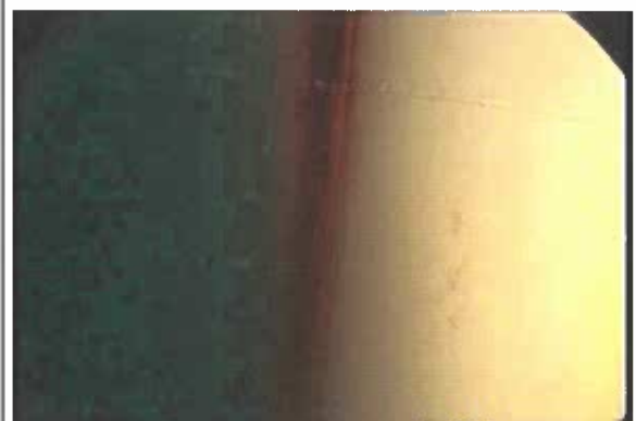
5:29 Staining on upper shell rings
