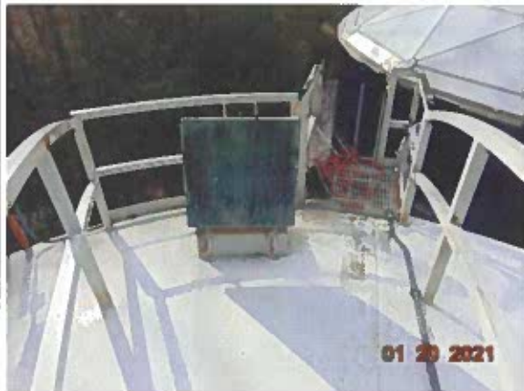
#19 Overview of roof access hatch and tank ladder
