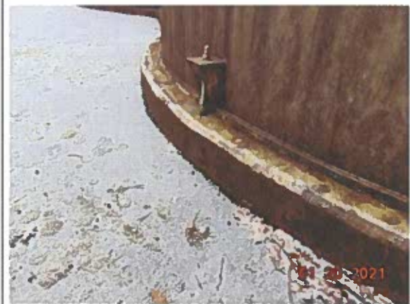
#9 Typical view of tank foundation
