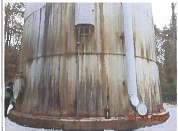
#12 Tank ladder height from grade
