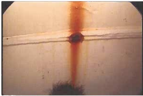
6:52 Brushed corrosion cell
