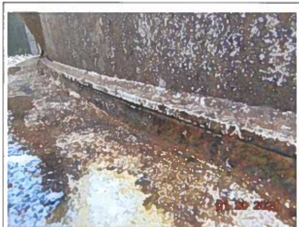
#10 Typical view of chime grouting
