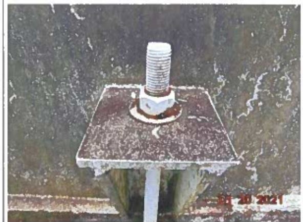
#11 Typical view of tank anchor
