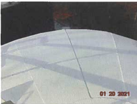
#15 Typical view of roof plates
