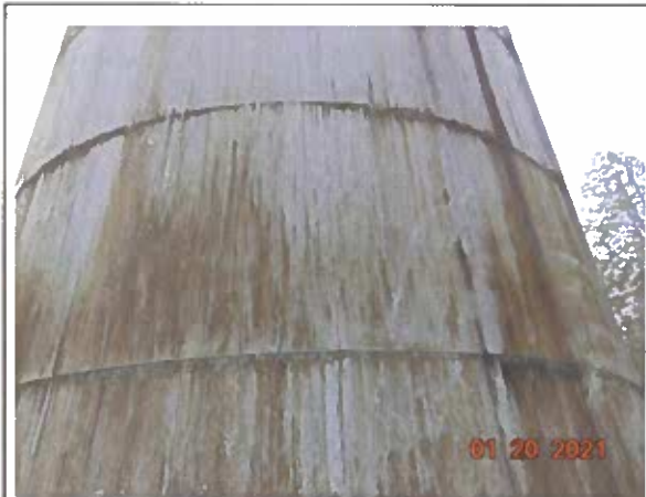
#7 Typical view of lower shell rings
