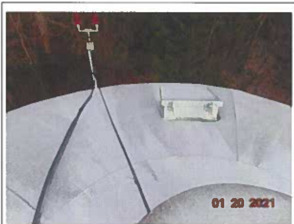
#16 Secondary roof hatch
