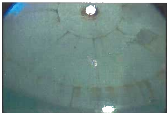
2:24 Interior view of roof vent
