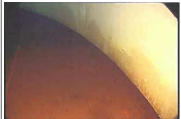
12:39 Typical view of tank floor
