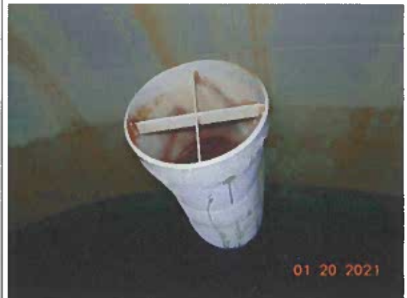
#22 Interior view of overflow weir funnel
