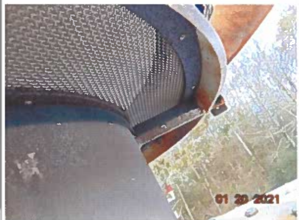
#18 Roof vent with intact fine screen
