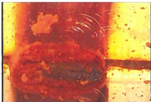
11:06 Exposed weld seam
