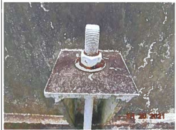
#11 Typical view of tank anchor
