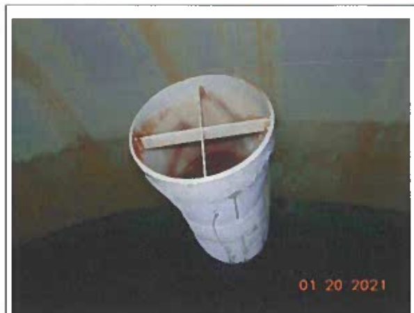
#22 Interior view of overflow weir funnel
