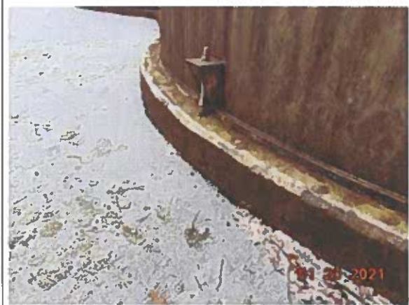
#9 Typical view of tank foundation
