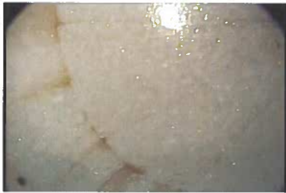
0:58 Typical view of roof plates
