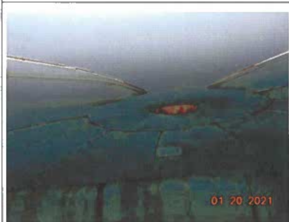
#21 Interior view of roof
