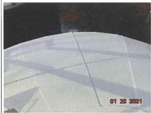
#15 Typical view of roof plates
