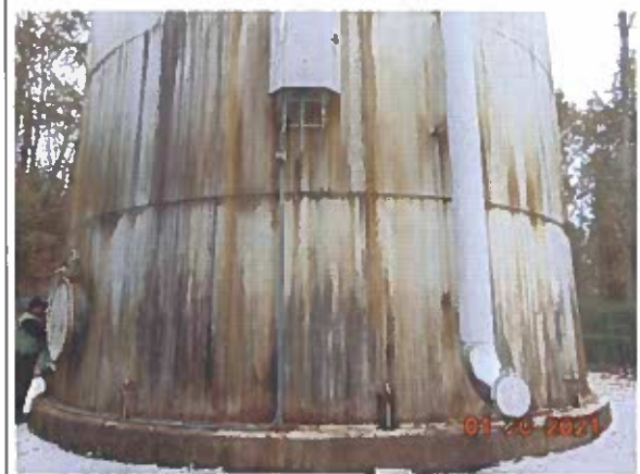
#12 Tank ladder height from grade
