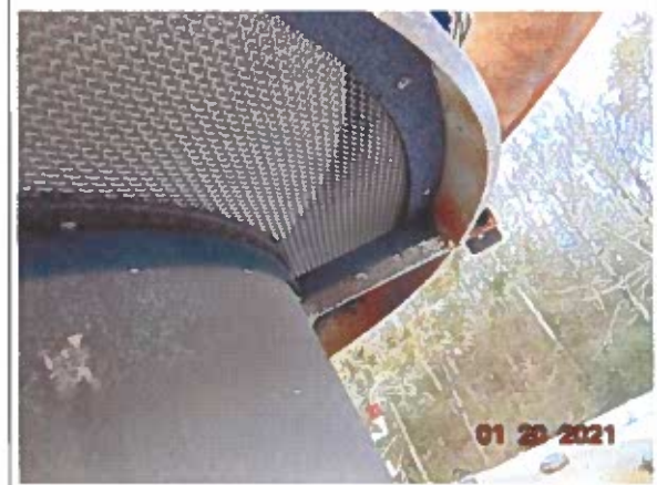
#18 Roof vent with intact fine screen
