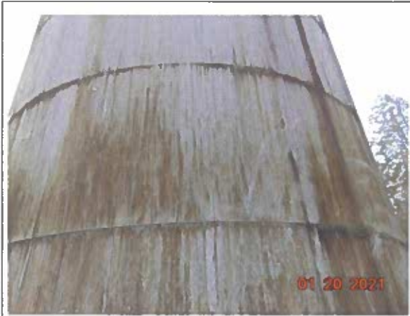
#7 Typical view of lower shell rings
