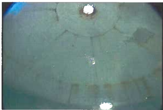
2:24 Interior view of roof vent
