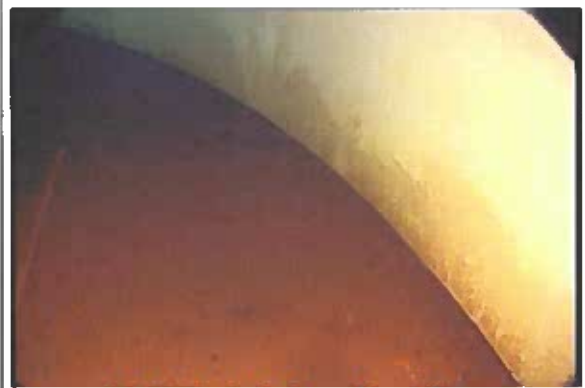
12:39 Typical view of tank floor
