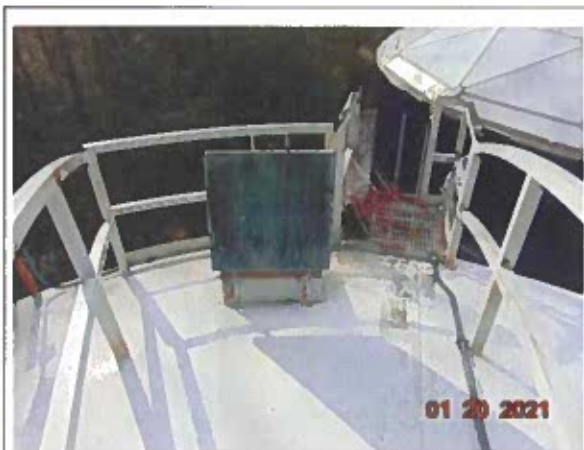
#19 Overview of roof access hatch and tank ladder
