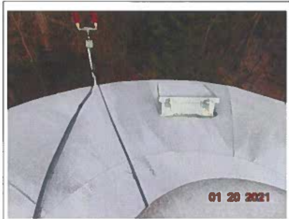
#16 Secondary roof hatch
