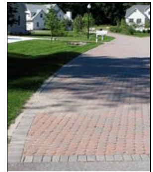
Pervious Pavers At Jordan Cove Site
