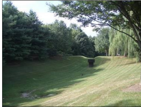
Water Quality Basin
