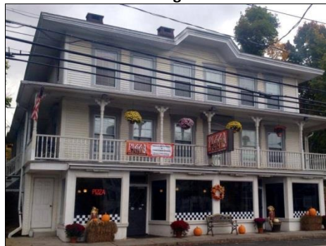
Mixed-Use building on Main Street
