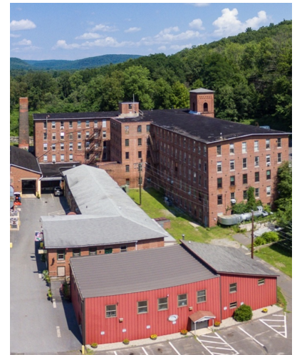
Existing Adaptive Reuse- New Hartford Business Park hurleybusinesspark.com
