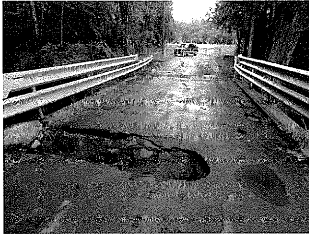
Current condition – November 2013
