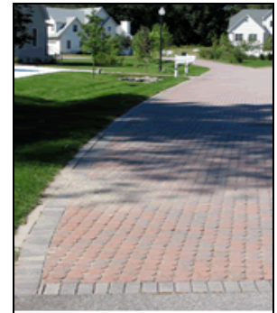
Pervious Pavers At Jordan Cove Site
