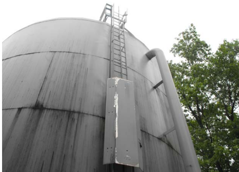
002.JPG 04/15/2010 Exterior shell ladder equipped with rail climb and anti-climb.
