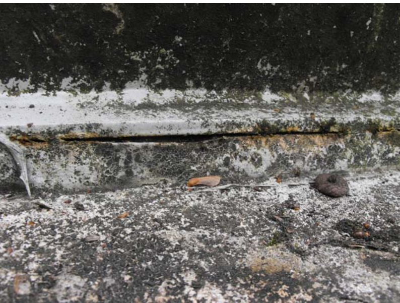
009.JPG 04/15/2010 Slight grout separation area under chime plate.
