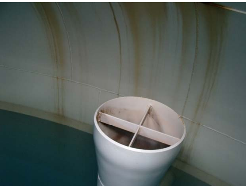
023.JPG 06/03/2009 Interior overflow pipe
