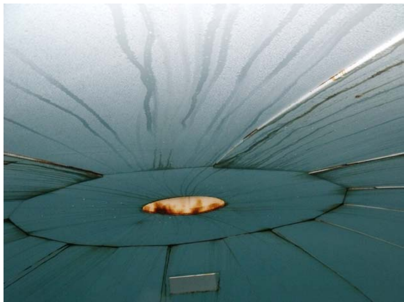
020.JPG 06/03/2009 Interior dollar plate with edge corrosion
