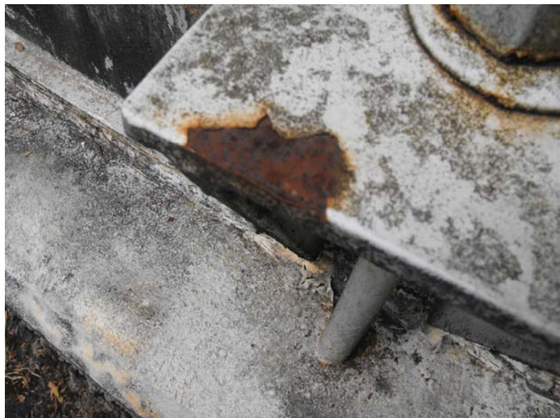
006.JPG 04/15/2010 Closeup of spot corrosion area on anchor chair.
