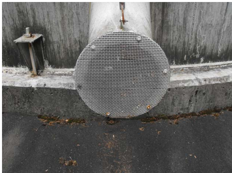
004.JPG 04/15/2010 Fine screening on overflow outlet.
