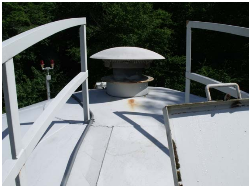
014.JPG 06/03/2009 Roof safety railing and center roof vent
