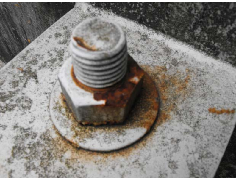
007.JPG 04/15/2010 Surface corrosion on anchor nut and bolt.
