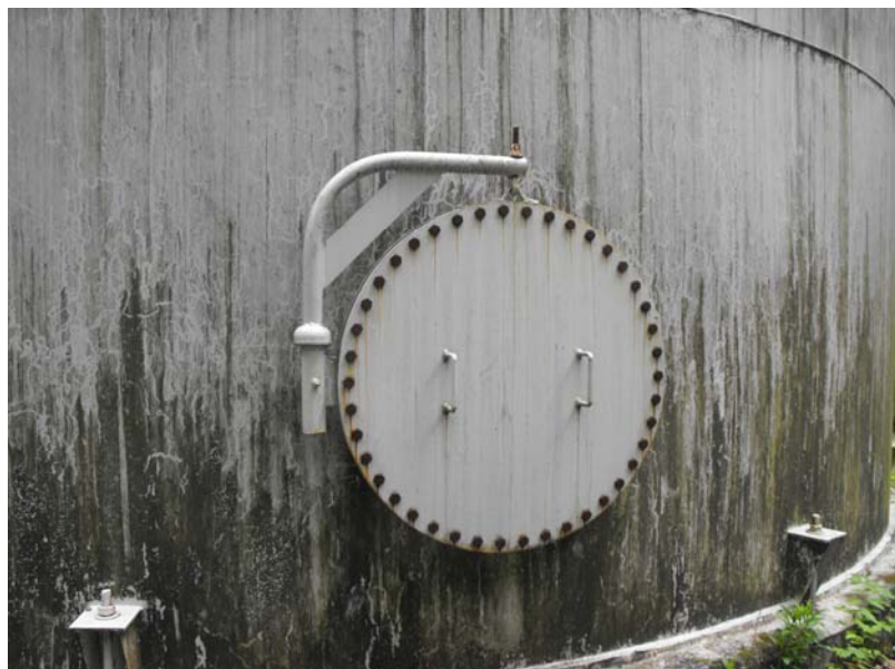
008.JPG 04/15/2010 36-inch round shell access hatch (1 of 2)
