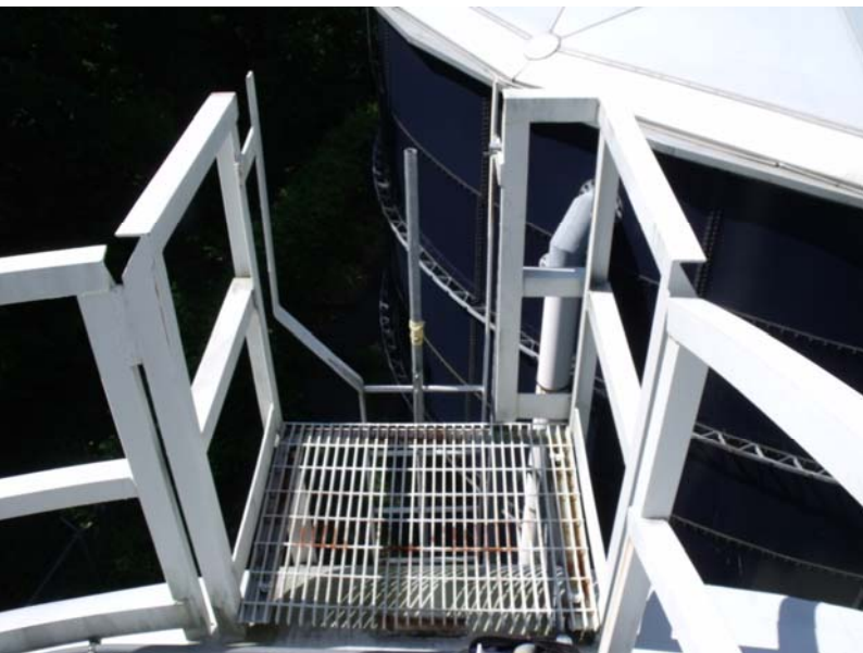
013.JPG 06/03/2009 42-inch roof railing equipped with mid-rail and toe kick.
