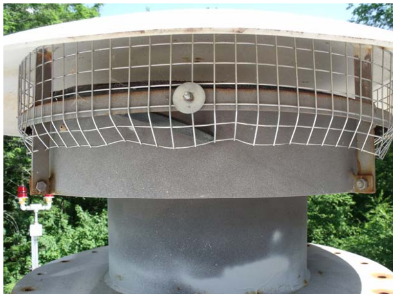
016.JPG 06/03/2009 Coarse rscreen outside with fine mesh under cap. All bolts replaced at time of inspection.
