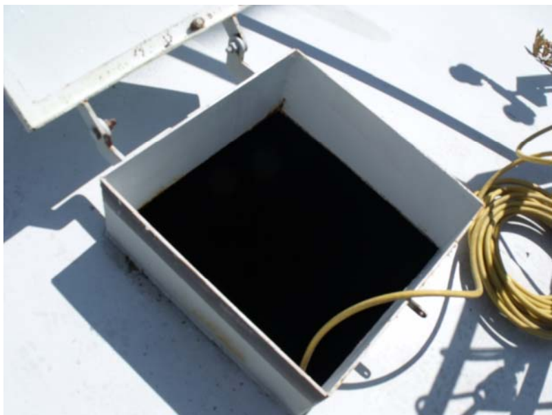
012.JPG 06/03/2009 24-inch roof hatch.
