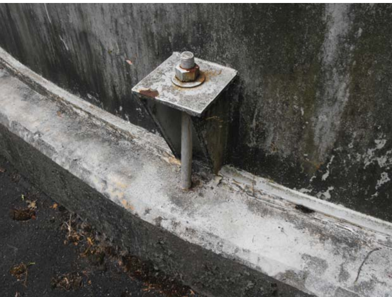
005.JPG 04/15/2010 Spot corrosion area on anchor chair.
