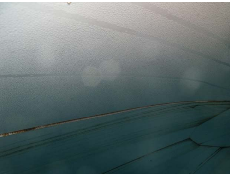
021.JPG 06/03/2009 Edge corrosion on roof plate seams
