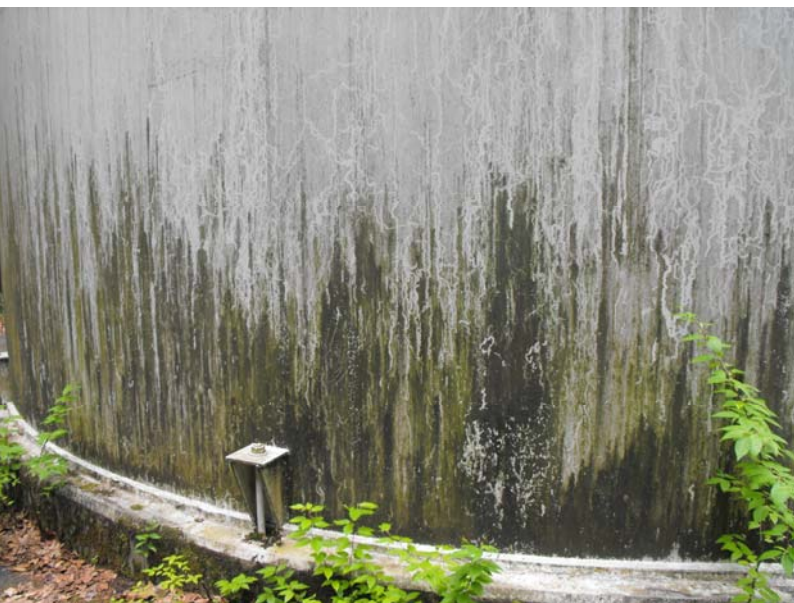
011.JPG 04/15/2010 Moderate mildew staining on tank base.
