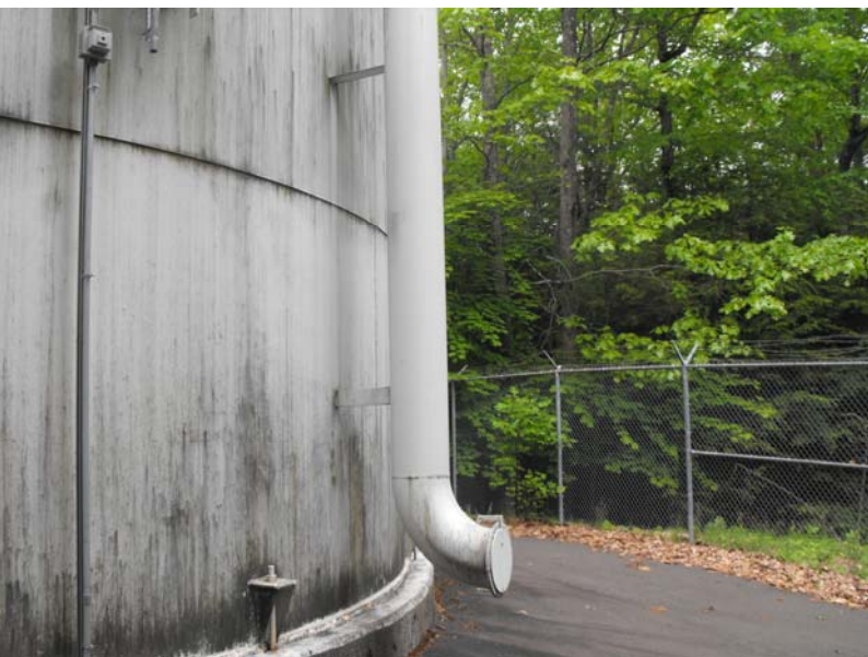
003.JPG 04/15/2010 Overflow outlet equipped with flapper valve
